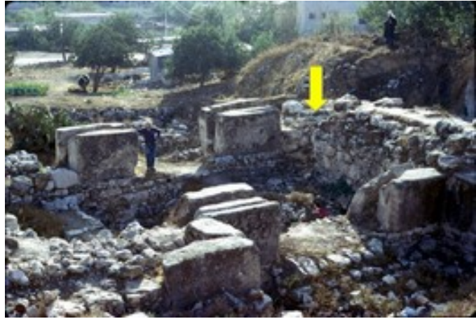
Figure 21: East gate of Shechem. Arrow shows doorway to stairwell leading to second story. Van and Anita Parunak, Nov 1974
