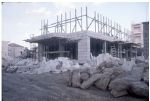
Figure 11: Pre-cut stones delivered to house under construction (Van and Anita Parunak, Apr 1975)
